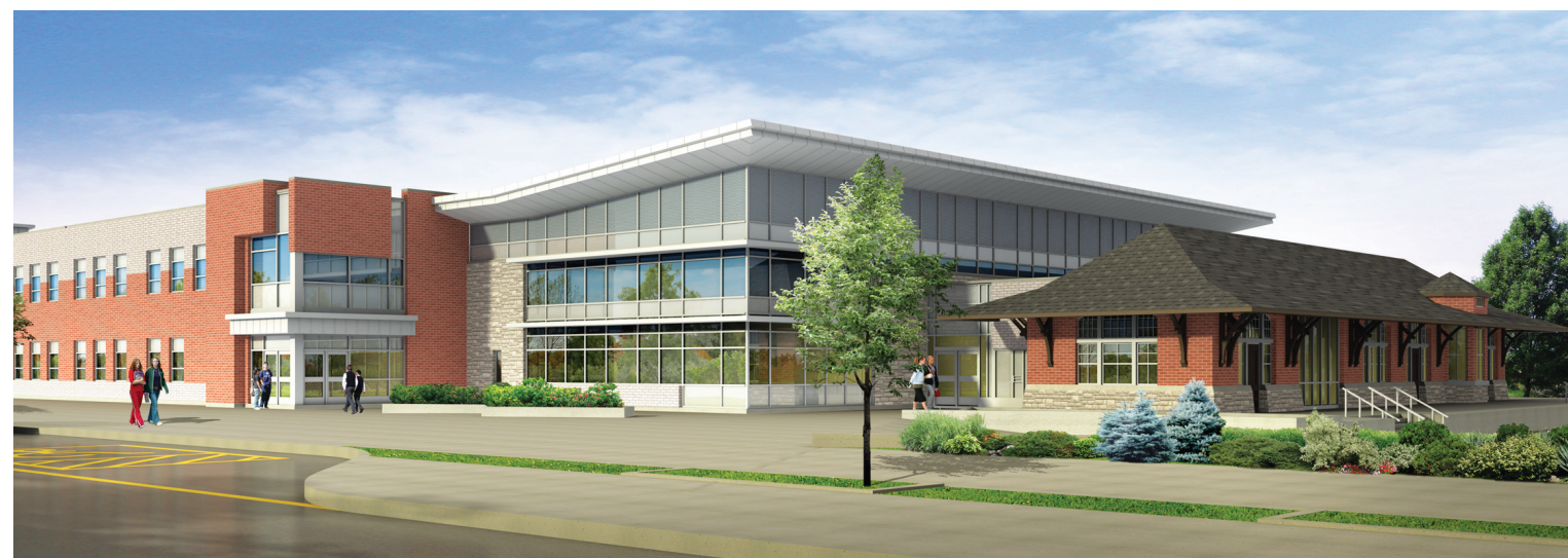
The Old CPR Station (far right) will be part of a new civic space (below centre and right) that includes a library and a school in Mount Pleasant Village.
