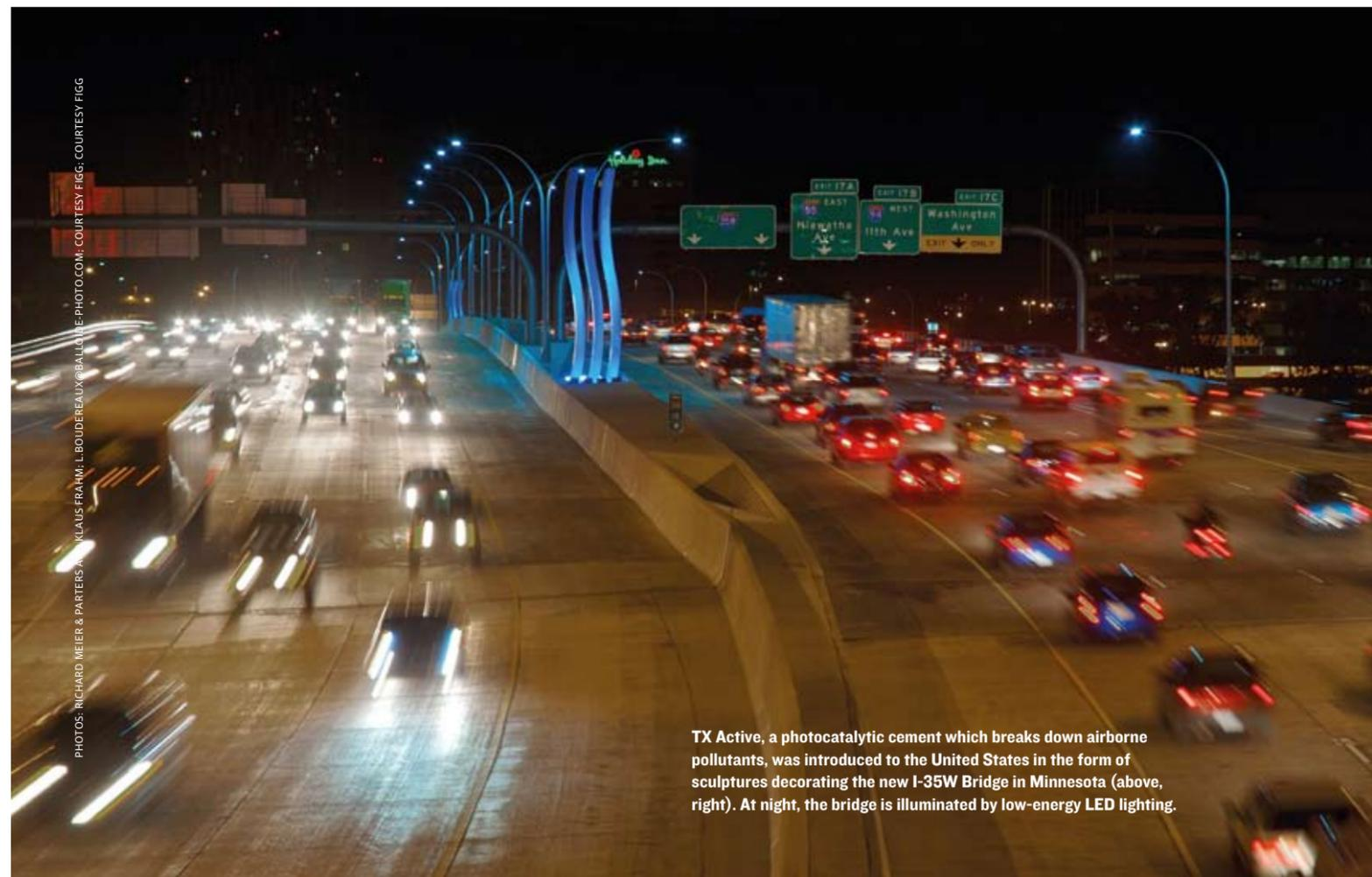
TX Active, a photocatalytic cement which breaks down airborne pollutants, was introduced to the United States in the form of sculptures decorating the new I-35W Bridge in Minnesota (above, right). At night, the bridge is illuminated by low-energy LED lighting.
