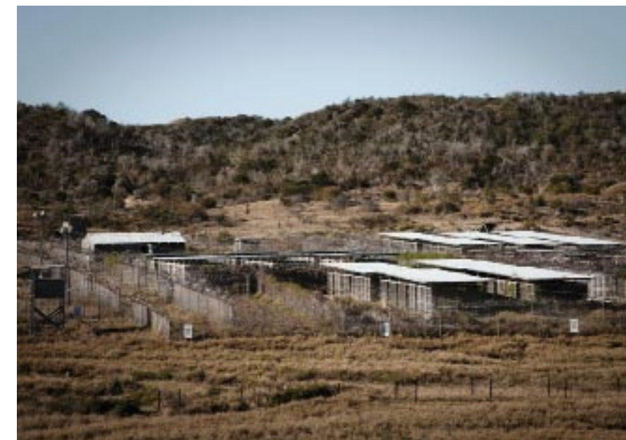
RAT-RUN: OVERGROWN AND DESERTED, CAMP X-RAY IS LEFT TO DECAY
