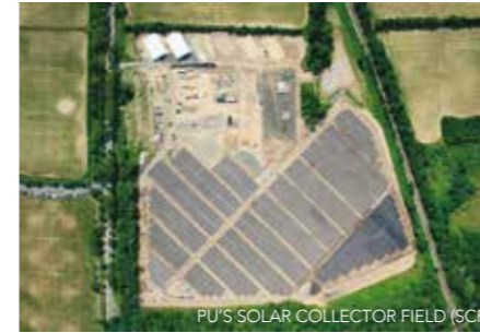
PU'S SOLAR COLLECTOR FIELD (SCF)
