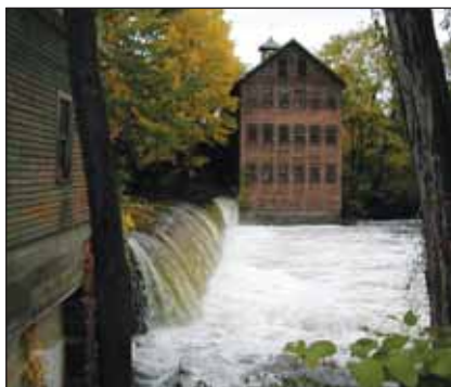
Many of the 2800 dams in Massachusetts have been labeled unsafe.
